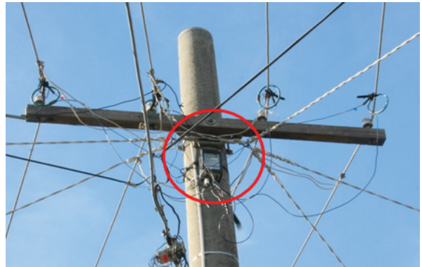
Fig. 4. Data loggers Records Voltage and Current parameters on the LV backbone
